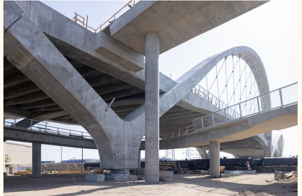
6th Street Viaduct, Los Angeles. Ø2 m, pendulum legur.
